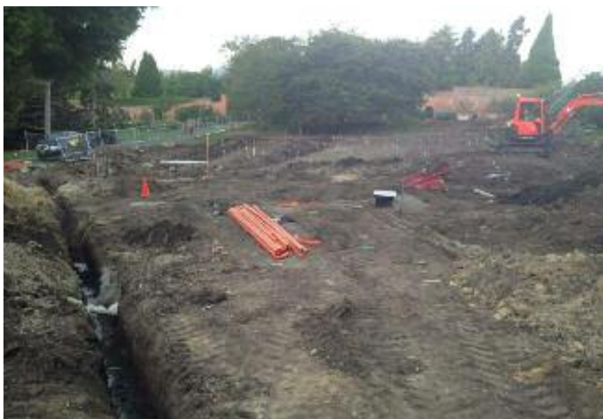
Work underway on the RTBG site
